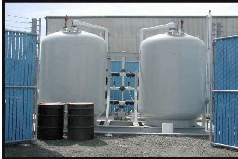
Two 2,000-pound liquid-phase granular activated carbon units.
